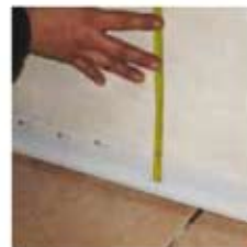
4 Measure the distance between the two profiles and cut the roll of T-Kone Plaster in equal measure
