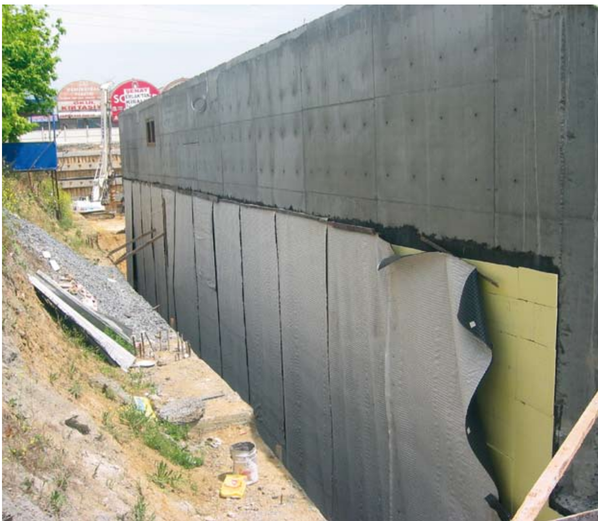
Mechanical protection of the waterproofing and drainage realised with T-Kone G Drain
