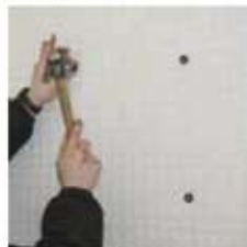
5 Fix T-K Plaster to the wall using T-Plug and T-Nail
