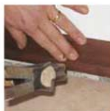
8 Position both below and above the skirting board
