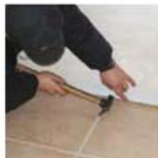
3 Fix T-Kone Plaster Profile “aligned” to the base and top of the wall using the provided nails
