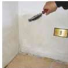
1 Clean the surface using a metal brush
