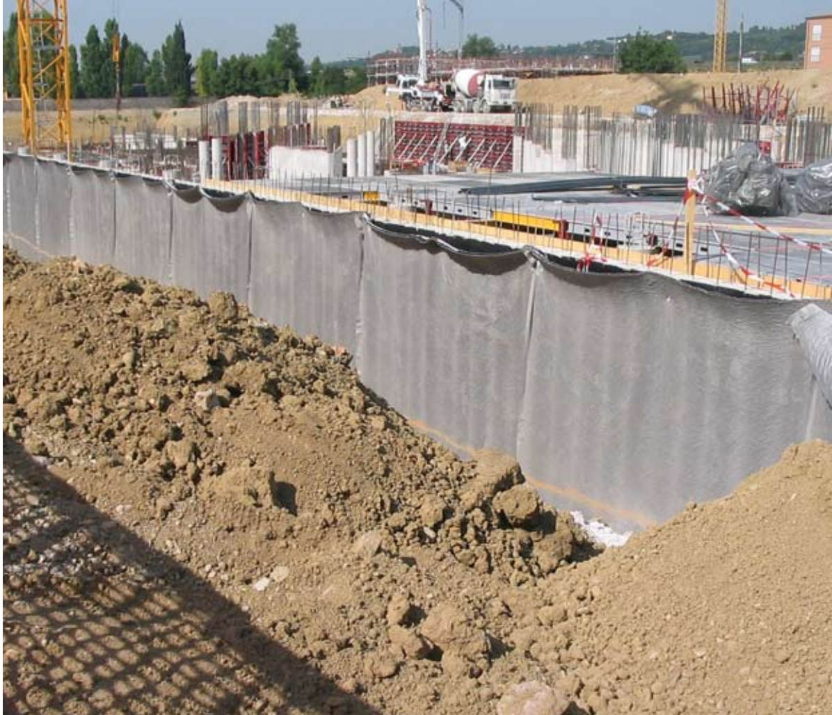
Mechanical protection of the waterproofing and drainage in correspondence of foundations of a shopping centre realised with T-Mix Drain 20
