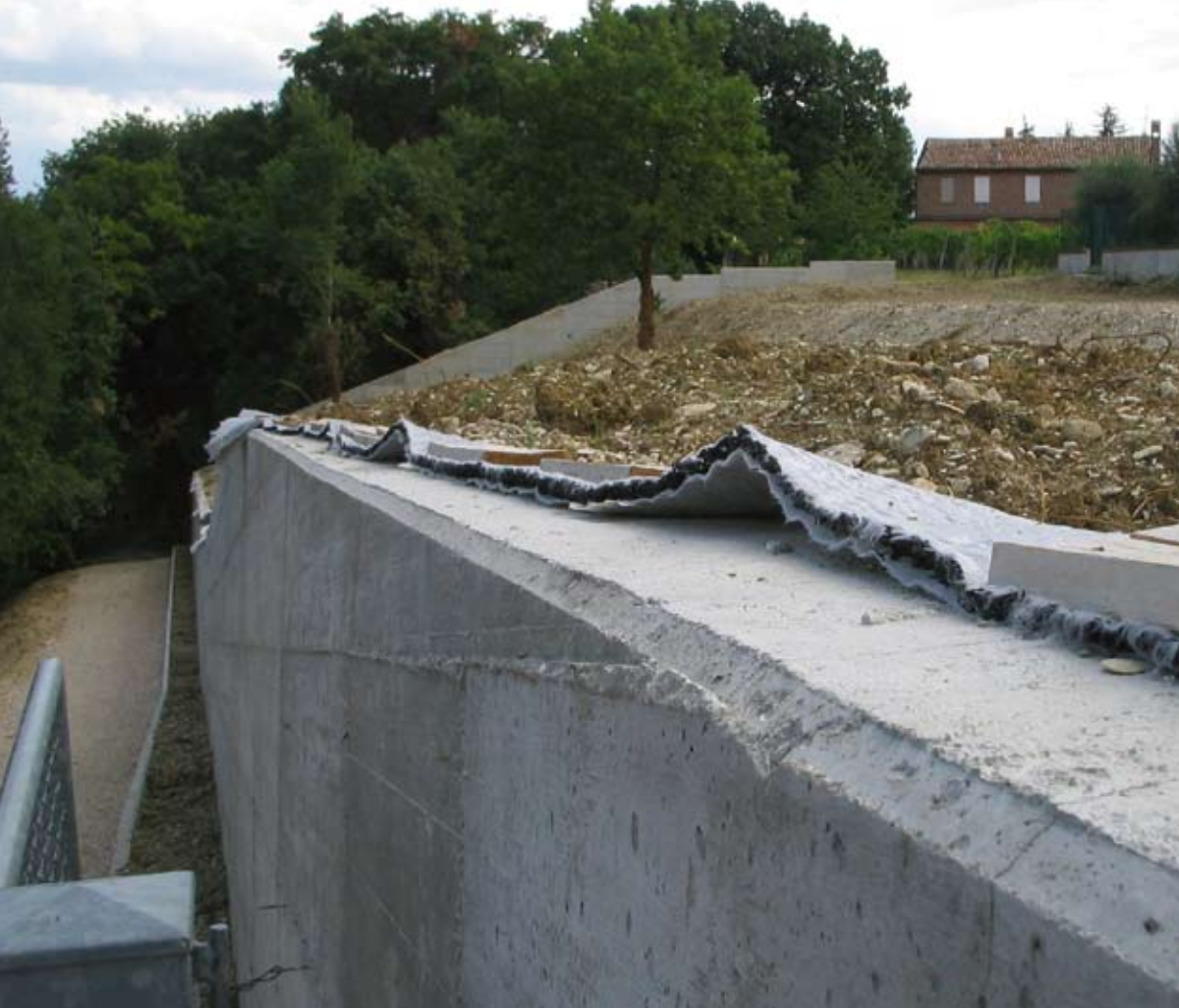
Mechanical protection of the waterproofing and drainage in a wall against earth realised with T-Mix Drain 20
