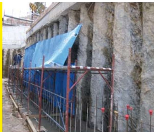
Waterproofing, drainage and disposable casing in a foundation realised with T-Mix Drain 20 WP
