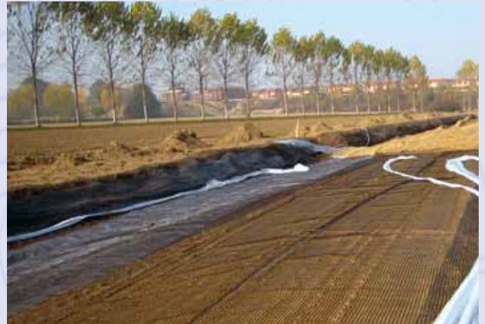
Application of the geogrids as road base reinforcement
