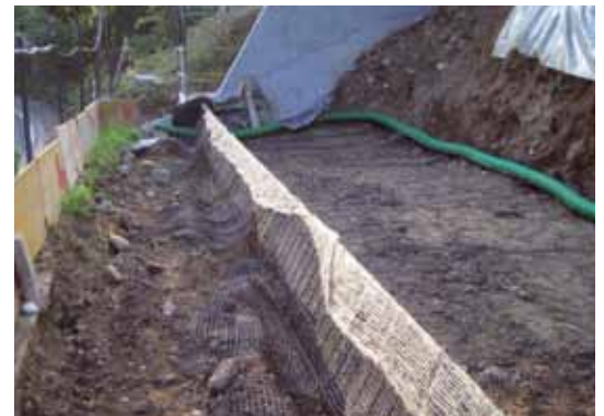
Particular of the drainage behind the work at the start of laying the reinforced earth system. The drainage collector is based at the bottom of the basement.
