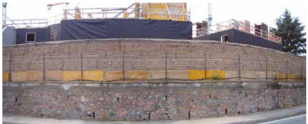
Particular of the drainage behind the work at the start of laying the reinforced earth system. The drainage collector is based at the bottom of the basement.
