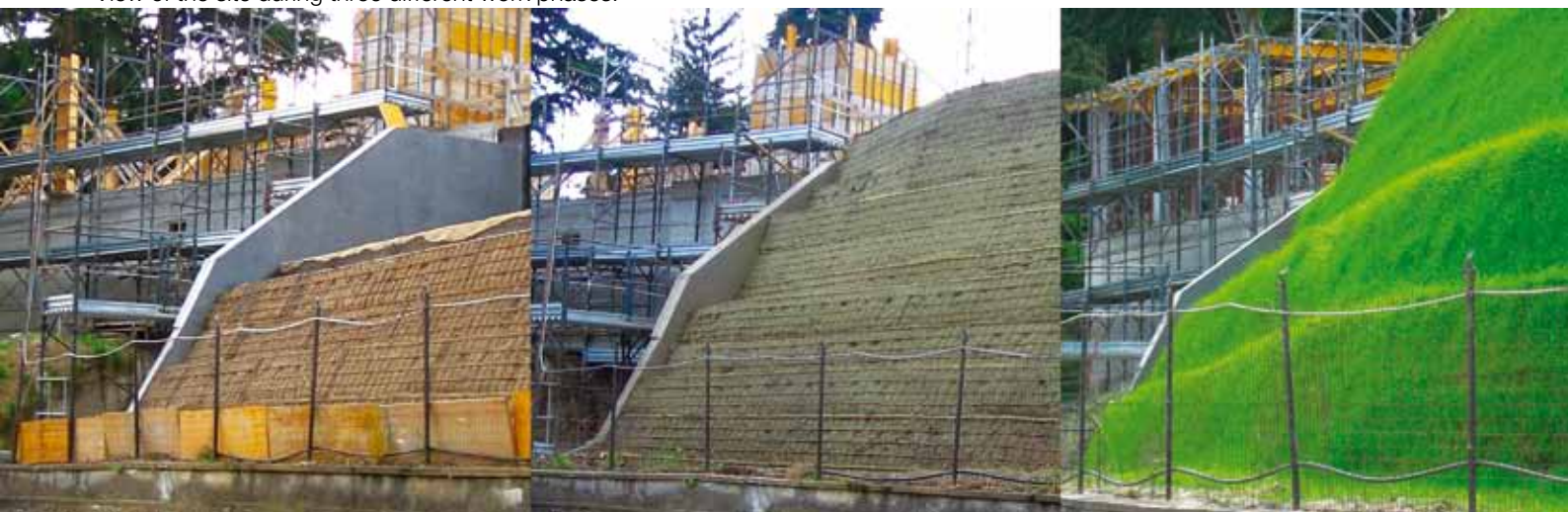
View of the site during three different work phases.
