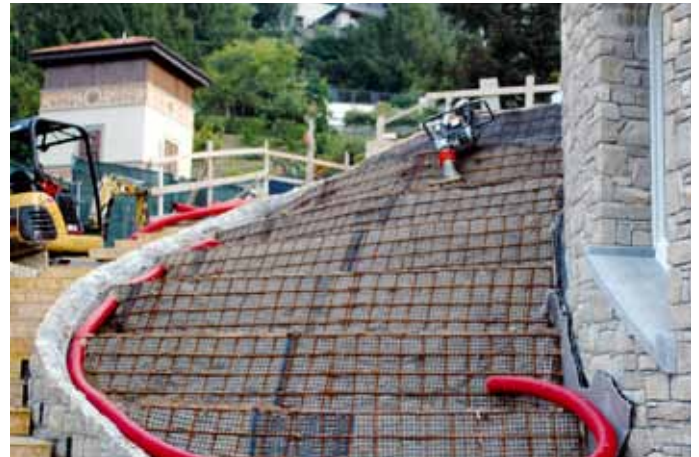
Reinforced earth in the private building sector
